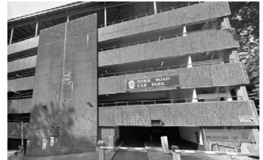
York Road Car Park
