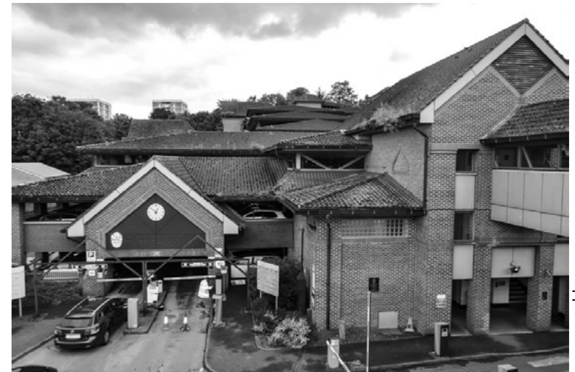
Farnham Road Car Park
